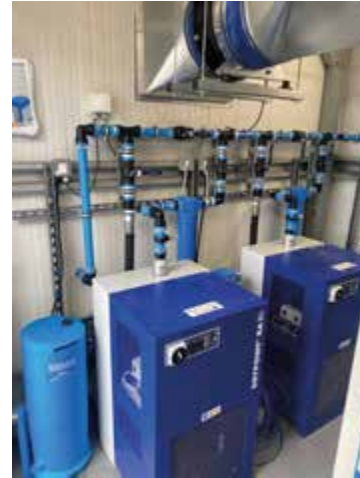
Twin Almig F-Drive 37 (37kW/50hp) compressor system operating in duty rotate. Factory fitted with Almig heat recovery system.
