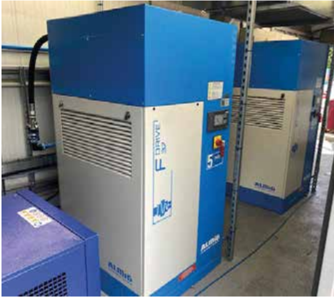
Twin Almig F-Drive 37 (37kW/50hp) compressor system operating in duty rotate. Factory fitted with Almig heat recovery system.
